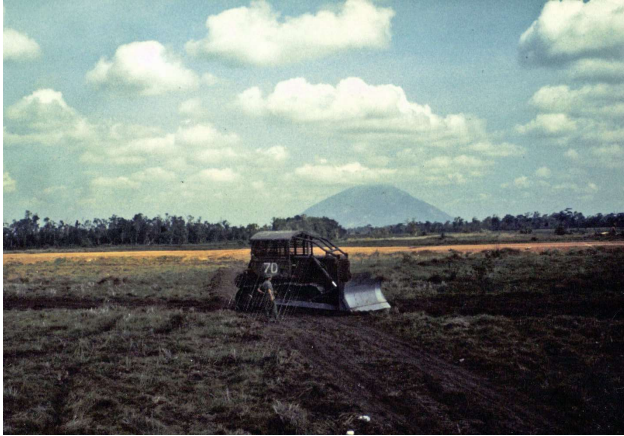
Roam Plows in the Jungle all done w nui ba dinh.jpg | Typically the plows would clear a wide zone around roads to prevent ambushes. This once was lush jungle and deny cover to enemy troop movements. (1429x997)
