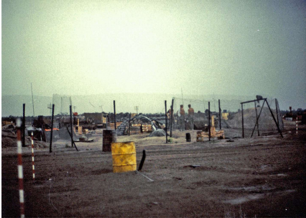
Company B basecamp near Chu Chi.jpg | We used chain link fencing strung up between steel fence stakes as an RPG screen. Notice the candy gains to the left of the picture. Those are mortar sighting stakes for use on night mortar fire missions. (1426x1020)
