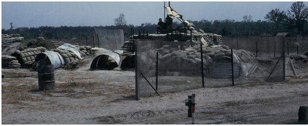
Company sized forward basecamp somewhere outside of Trang Bang, off the road to Dau Tieng 2. JPG | Typical fire support base. sleeping and shooting "tunnels" were made from 1/2 drain culverts (see some uncovered in the background). Sand bags covered the culvert halves and a wall was built in front with a window for firing from. A back wall was built to protect from incoming mortars and out going artillery. (1789x718)
