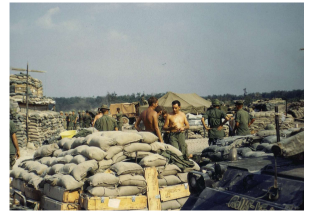
Hard Spot outside of the Ben Cui with lots of sandbags.jpg | This was our "Hard Spot" just outside of Dau Tieng. Everything was layered in sand bags, and a 10 foot berm surrounded the entire complex. There was foo gas on every corner, each track pulled into a carve-out in the berm, and each track berm mounted a 50 cal along with its regular track mounted 50 cal. This was the most heavily sand-bagged and defended small forward base I was ever in. (1412x1003)
